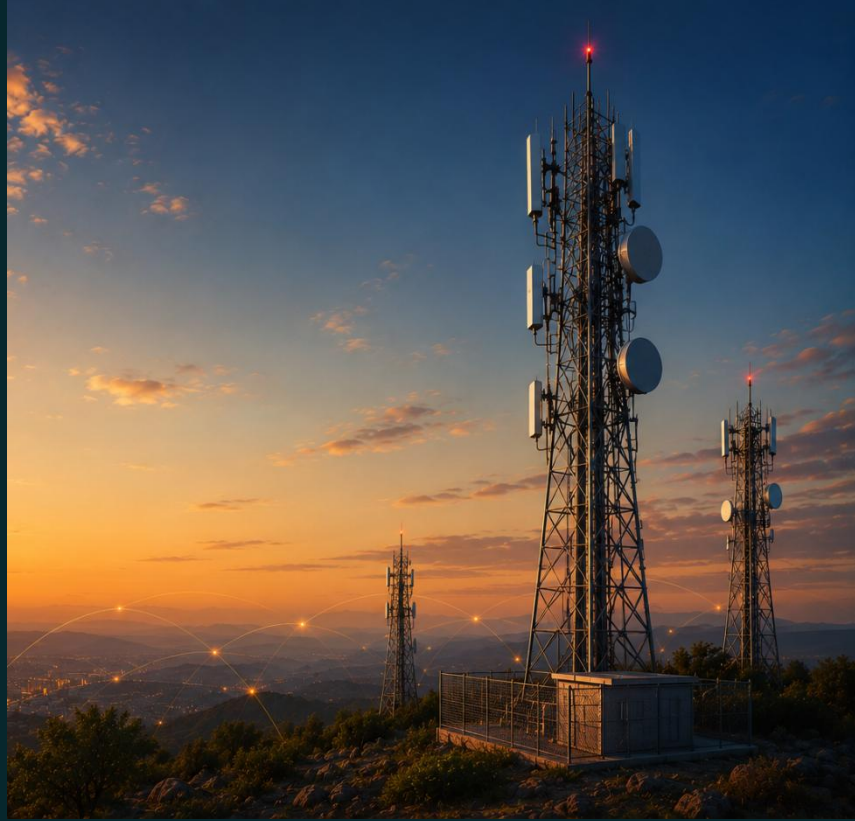
Phase 1: Offgrid Telecom Towers
